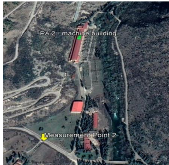
Figure 21: Position of the measuring position 2 at the Bogetići/Glava Zete site
