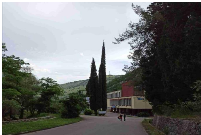
Figure 2. Location 2- Mechanical building of HPP Perućica
