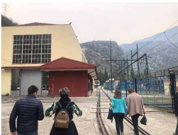
Machine building(powerhouse) of HPP Perućica
