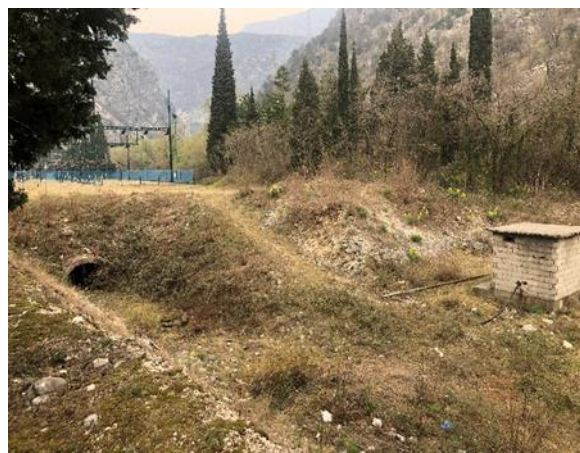
Outflow canal for unit 8
